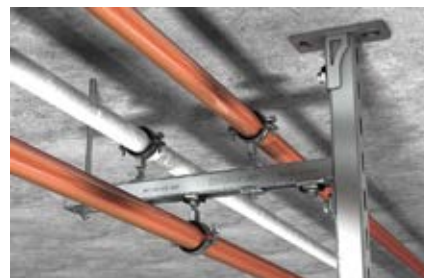
Cantilever construction with channel
